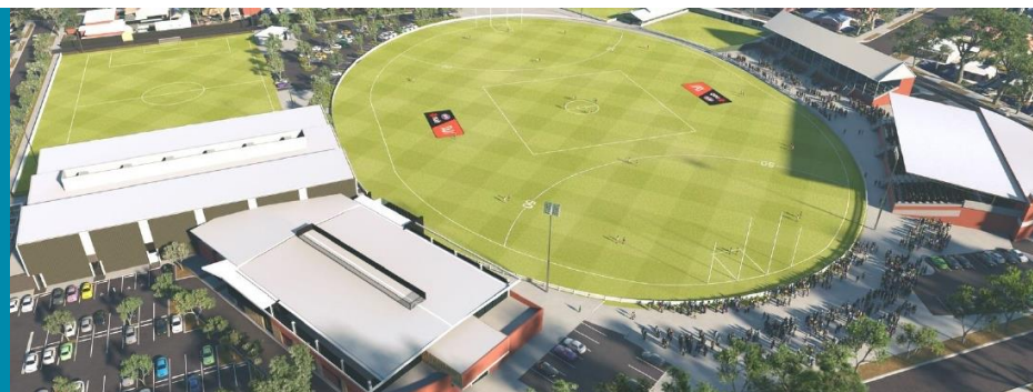
ALLAN SCOTT HQ/MG HIGH PERFORMANCE CENTRE
